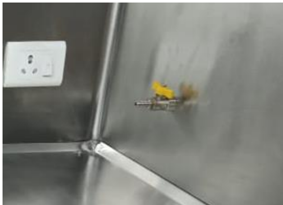
ELECTRICITY SOCKET WITH SWITCH & VACCUM TAP
